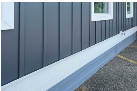
PVC TRIM BOARDS WITH BOARD & BATTEN SIDING
